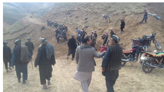
Community members working during the road construction in Kawlian Valley, Pulicharagh district
